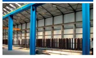
GCA provided a complete design and project management service for the extension of a factory to provide additional work space for Eggleston Brothers Steel Fabricators. The provision of new working space, as well as overhead gantry cranes and storage areas, required a detailed assessment of the design loads, and the provision of an economic steel portal frame.
